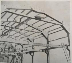
Fig. 1. Rigid frames for this 40x160-ft, building aid in supporting the second floor have gable roofs pitched one on eight by means of 11/2-in. dia, rod hangers. Gusset plates are of plywood and split and covered with the corrugated ring connectors are used.
