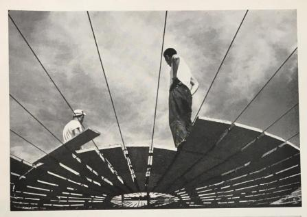
Miniature of Montevideo roof system 50' in dia., using 36 cables, was designed and built last summer in Columbia University camp at Litchfield, Conn., by architecture and engineering students under supervision of Bruno Funaro and Mario Salvadori. Compression ring is laminated wood stiffened by steel. Temporary overloading was with sandbags. Drainage here is simply into pool below open oculus; normally it would be handled by sump pump. Salvadori says snow and ice accretion would be no problem.
